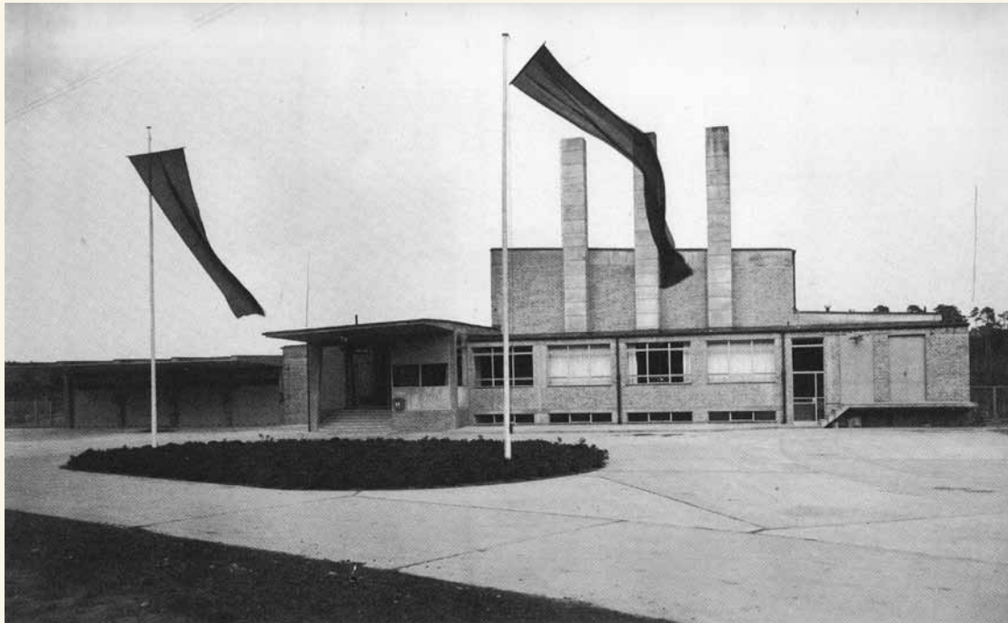
Hannes Meyer, Hans Wittwer and the Dessau Bauhaus building department: General German Trades Union school in Bernau, near Berlin, 1928-30. Meyer and Wittwer made the three chimneys of the oil-firing system the dominant motif of the school's entrance, leading one pupil to describe it as an "education factory". On the right, a loading ramp; left, garages.*
